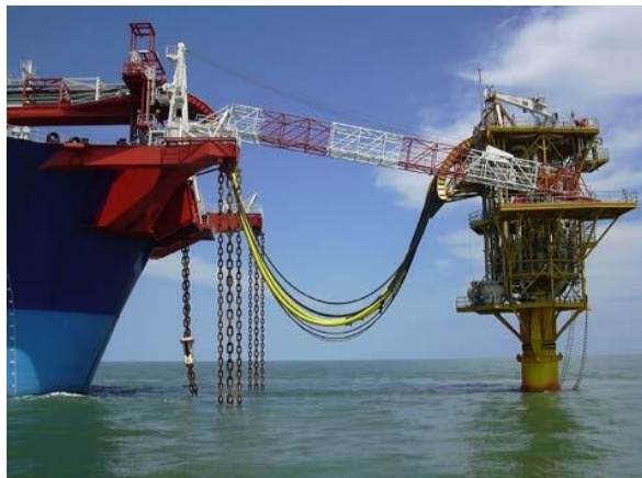
Figure 6: Platform loading arrangement (Source: APL)
