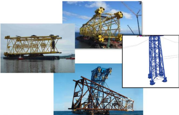
Figure 2-2: Typical 4- leg Jackets
